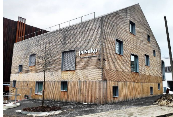
The year of construction 2020, photo 2021, Lithuania. The compass point also affects the progress of the graying process. The color can sometimes be partially or completely black. Momentary humidity conditions also affect the prevailing tone of shades. The installation direction also affects the speed of the process.
