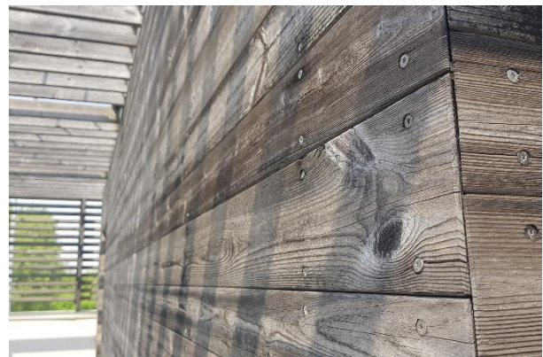
The year of construction 2009, photo 2019, Italy. Although the graying process has reached its end point, there are still shade variations in the surface according to the variation in the natural properties of the wood.
