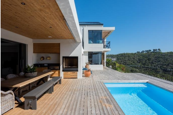
The year of construction and photo 2020, South Africa. The graying process has begun. The boards most exposed to UV radiation start first to fade. Part of them very uneven. This is due to the inherent properties of wood and their variation.
