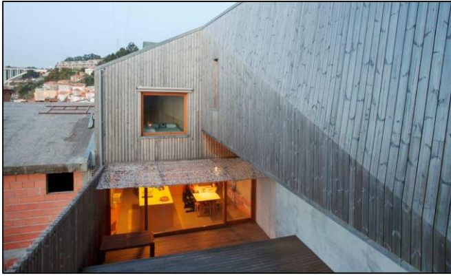
The year of construction 2015, photo 2019, Portugal. The surface has taken on a beautiful silver-gray hue. The part of the wall in the shady area has still retained its original, albeit faded tone.
