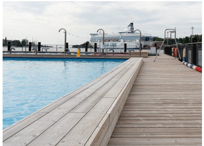
Allas Pool in Helsinki, 5 months after installation. Due to the even exposure to sunlight and moisture, the decking weathered rapidly to grey.
