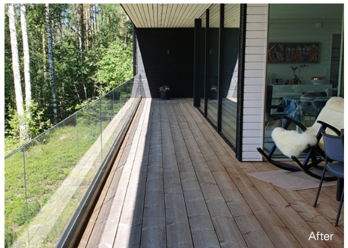
Lunawood decking immediately after installation and 2 years later. The decking in the sunny area has turned gray faster compared to the shaded area.
