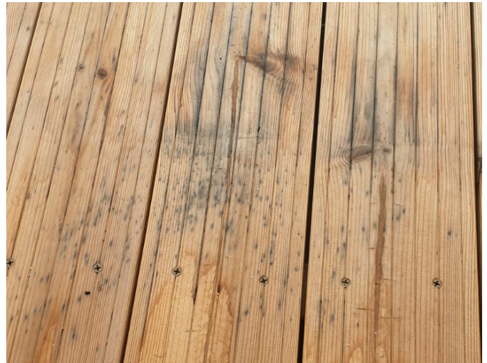
Impurities can cause small black spots on the surface of a decking.
