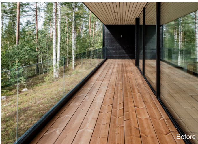
Lunawood decking immediately after installation and 2 years later. The decking in the sunny area has turned gray faster compared to the shaded area.
