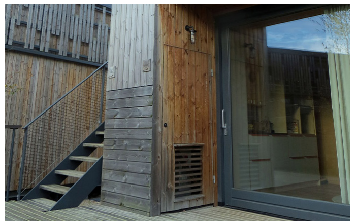
Cladding in the Netherlands two years after installation. The orientation of the building affects the progression of the greying process. The colour may sometimes appear partially or completely black. Humidity conditions can also influence the prevailing tone.
