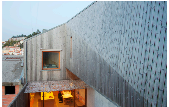
Cladding in Portugal 4 years after installation. The surface has taken on a beautiful silver-gray hue. ©Tiago Casanova
