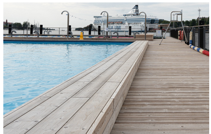
Allas Pool in Helsinki, 5 months after installation. Due to the even exposure to sunlight and moisture, the decking weathered rapidly to grey.
